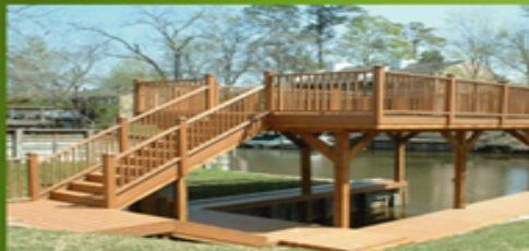
CPPC made Outdoor Structure
